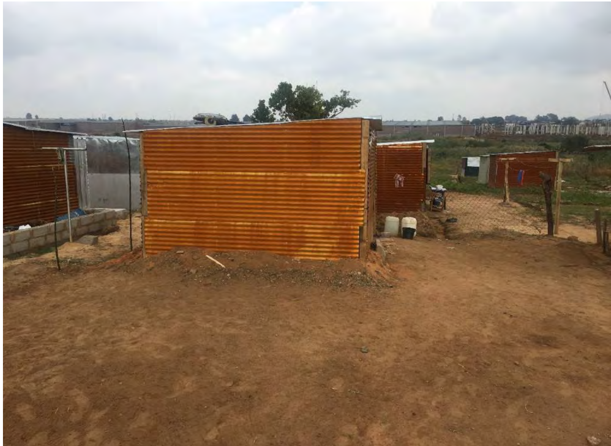
Images above: The new shack has a concrete floor
