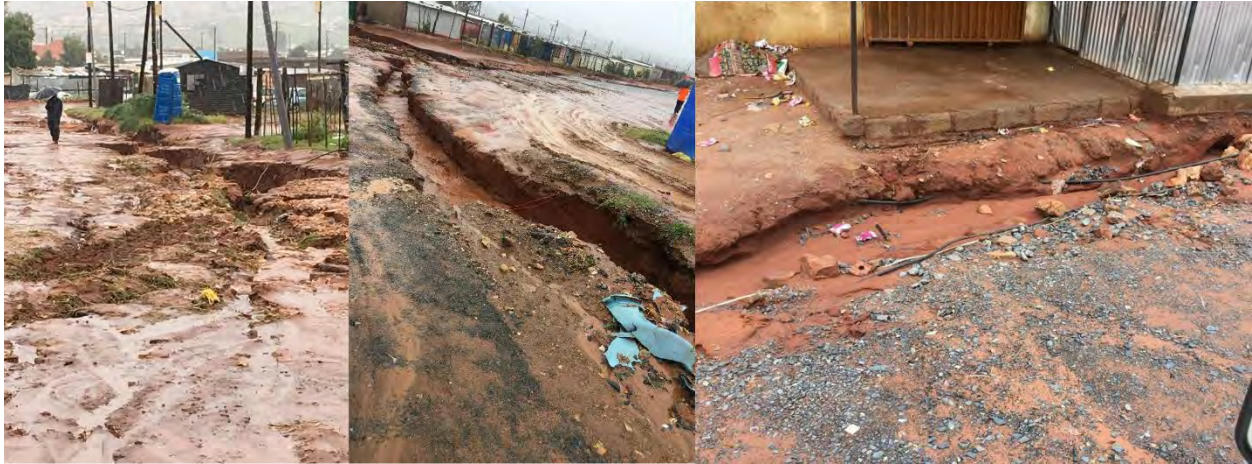
Images above: Since there is no proper drainage system, when it floods in Mamelodi, there are large gullies formed by the eroding water
