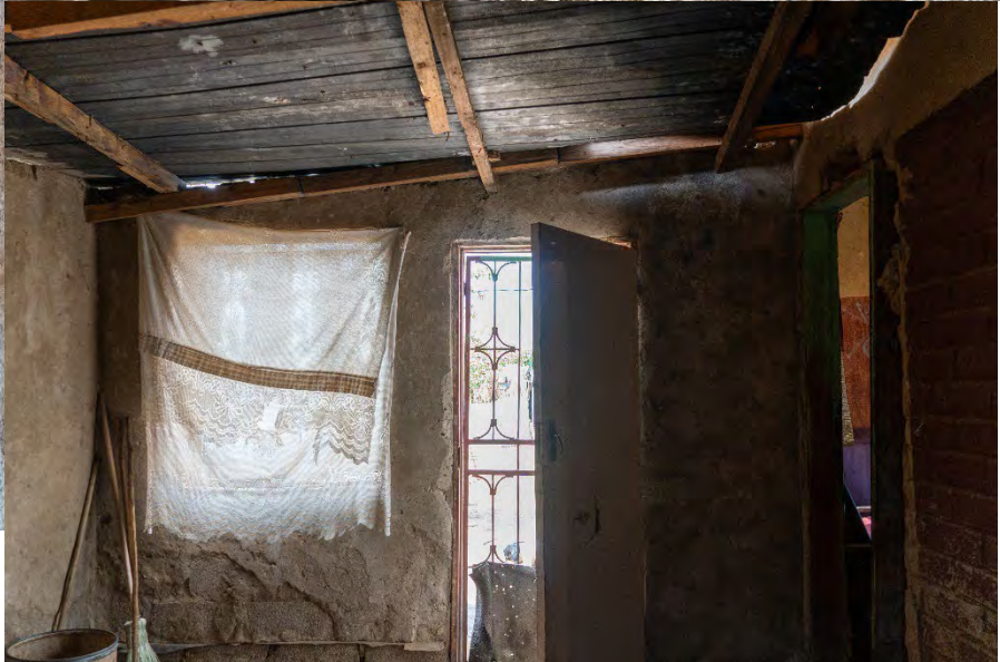
Images above: Various images of the inside of the new section
