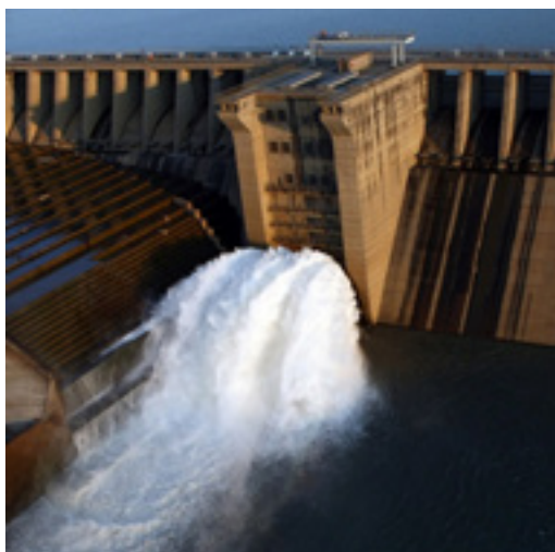
Potential to retrofit the Vaal Dam outlet works and generate a baseload energy of 4.4 MW.
