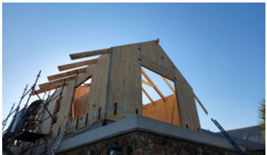
Vertical expansion of a residential building by Mass Timber Technologies.
