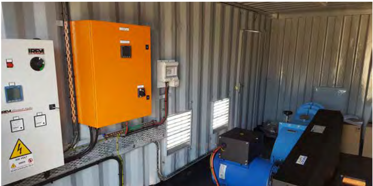
→ Installed turbine and control panel (Kwa Madiba).
