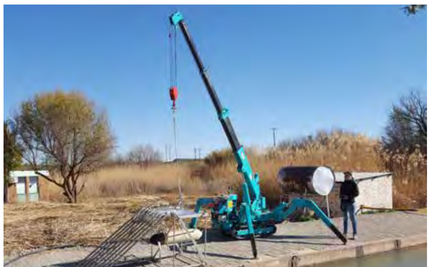
→ Installation of kinetic-type turbines in a canal.
