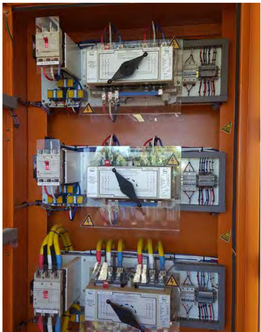
→ Section of the automatic changeover panel (Bloemwater).
