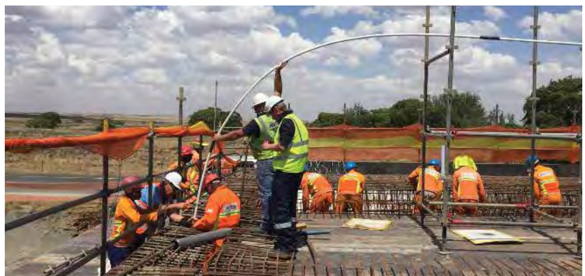
→ Installing the sensors on the Van Zylspruit Bridge.
