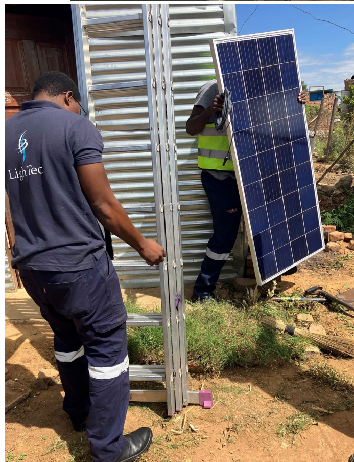
Technicians preparing to install solar panel on a shack
