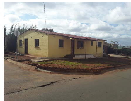
Thandanani Renovated Building
