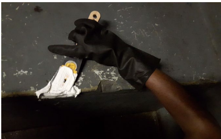
Photograph 4: Filling the holes in a wall with polyfilla
