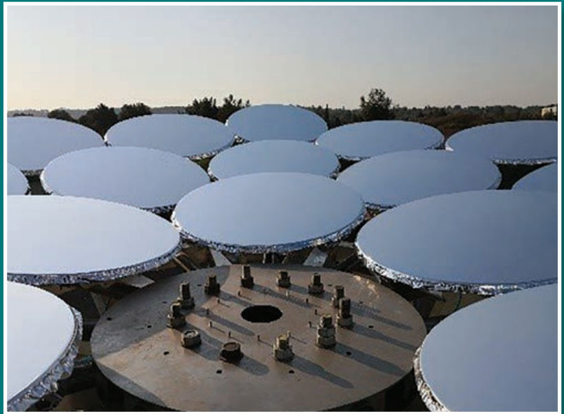
↑ Figure 2: The satellite dishes covered in reflective mirror membranes which can be adjusted through a vacuum to focus sun (or moon) rays onto a central collector.
