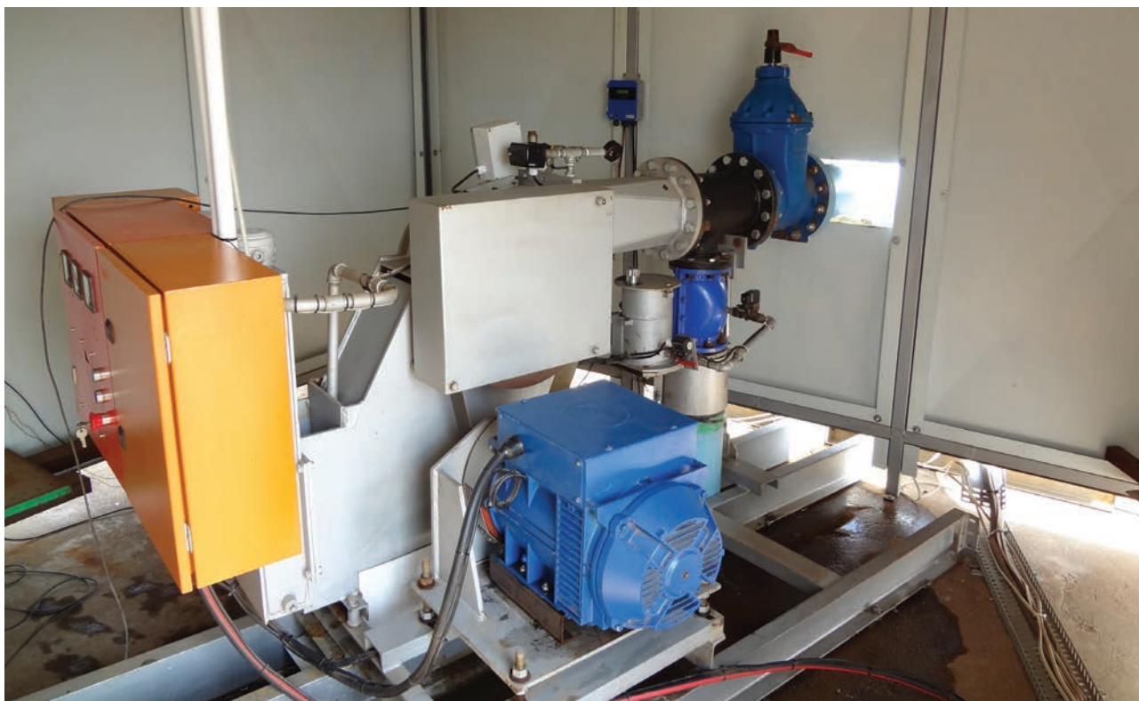
→ The conduit hydropower plant at the City of Tshwane, which generates power to be used for lighting, alarm systems and communication.
