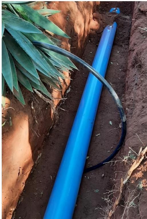
Figure 3.12. Photograph of one of the standpipes leading down to the level of the FO cable installed along the pipeline laid in Tom Jenkins Drive.
