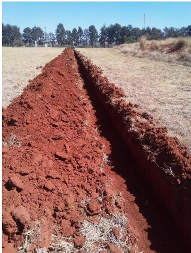
Figure 3.2. Standing point view of the trench prior to installation of the fibre optic cables.
