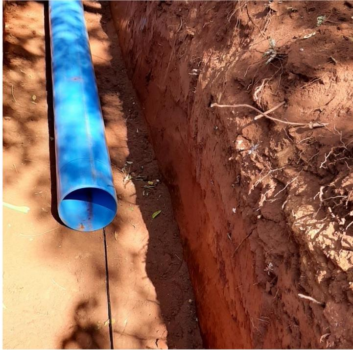
Figure 3.11. Photograph showing the position of the FO cable relative to the laid pipeline.
