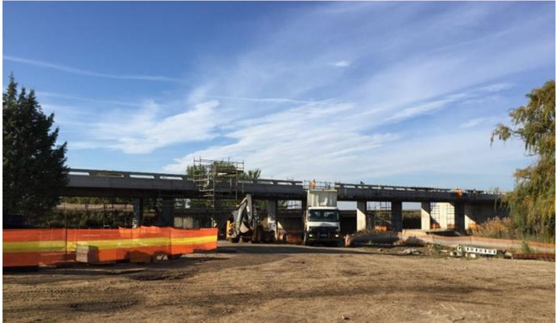
Figure 2.5: Van Zylspruit Bridge under construction (Skorpen et al. , 2016)
