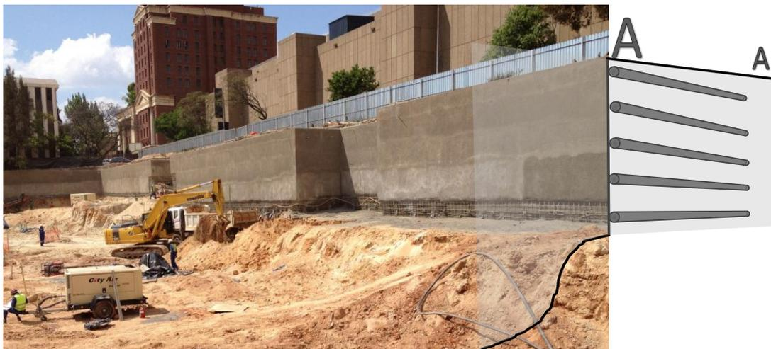
**Figure 4-5: Soil-nailed excavation during construction with cross-section A-A**
