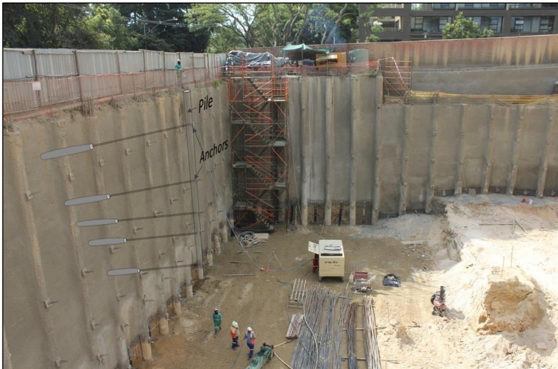
**Figure 4-36: Anchored excavation during construction**
