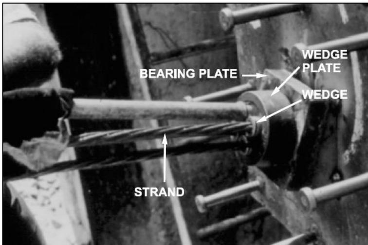
Figure 2-10: Anchor proximal end (FWHA, 1999)
