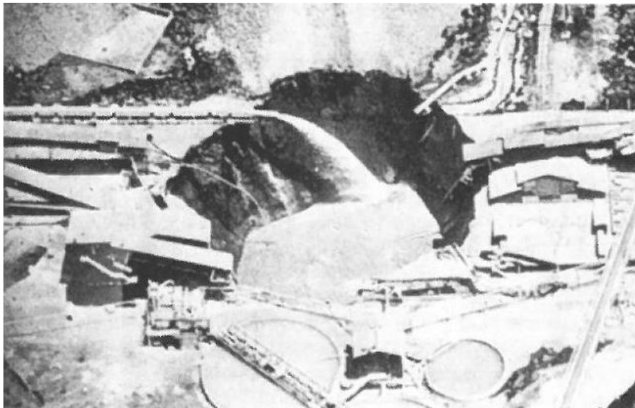
Figure 2-13: Sinkhole at the West Driefontein Mine, 1962 (Wagener, 1985)
