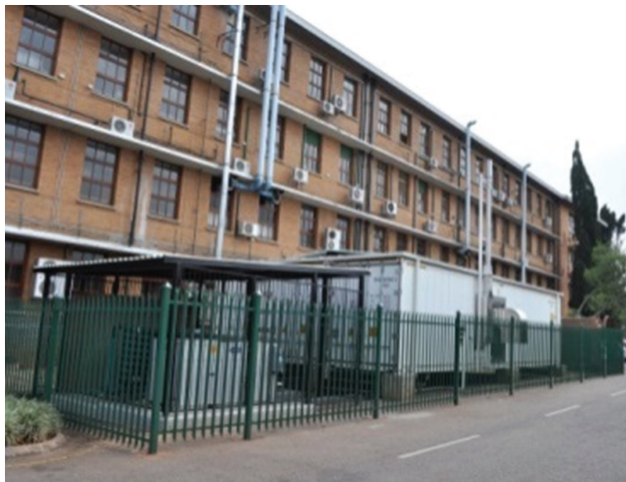
The completed laboratory adjacent to the Pathology Building. Air conditioning condensers and the effluent decontamination system are housed under a separate roof.
