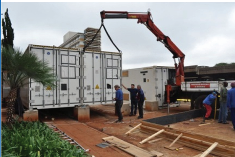
The containerized BSL-3 laboratory, erected on Prinshof Campus.
