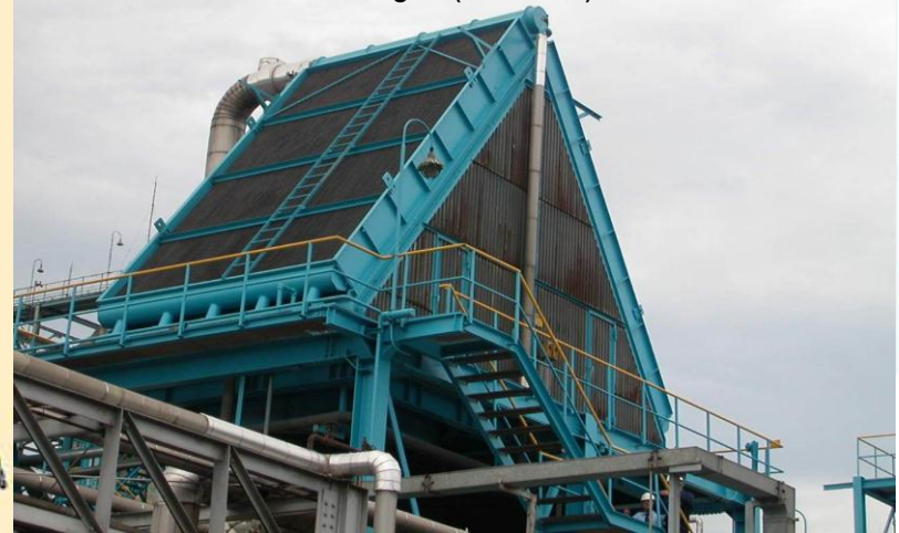
Air-cooled heat exchanger (2008 / 9)
